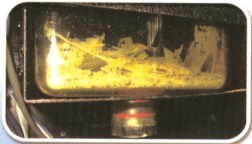
Encrusted with scale
